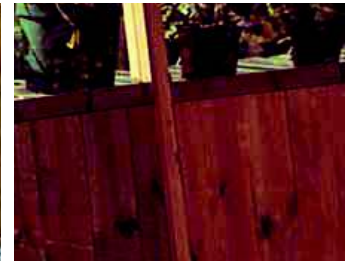
BOARDED PANELS - To conserve heat and provide shade.
