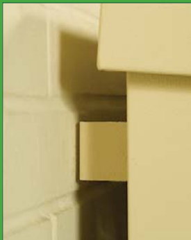
Mounting plate allows air flow to rear
